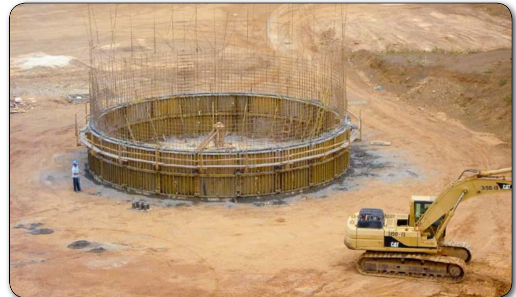
EFCO's REDI-RADIUS forming system is designed to form fixed or variable radius walls with diameters starting at 10'-0" (3 m) and greater.
