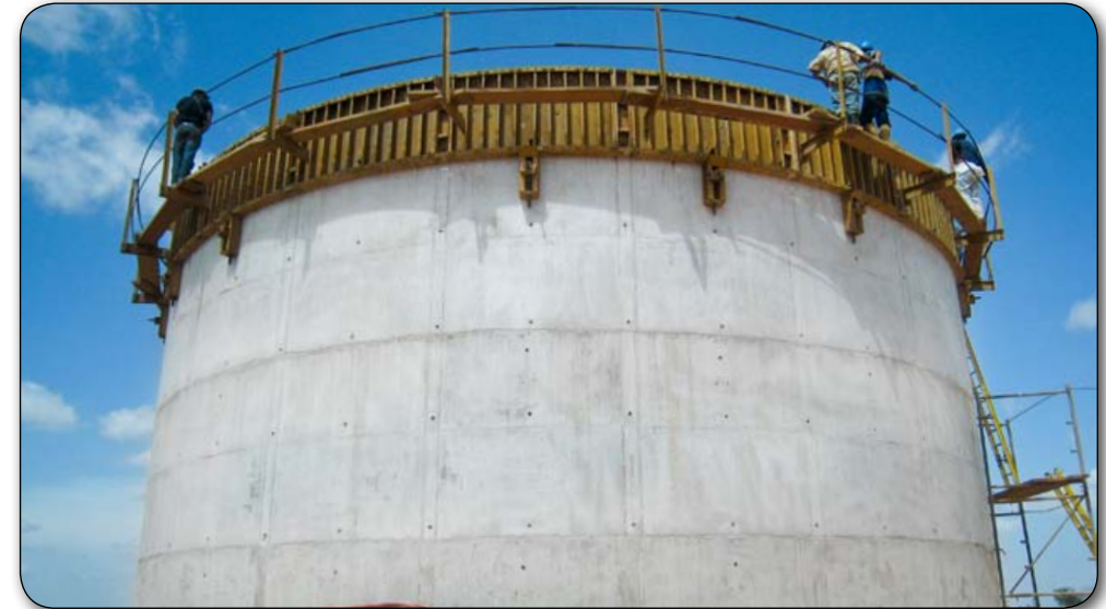
The all-steel REDI-RADIUS face sheet delivers a smooth continuous curved architectural concrete surface.
